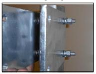
D) Insert ½" bolts through both sides of assembly
